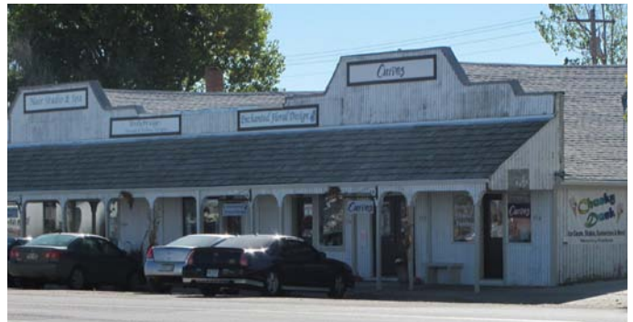
Figure 5.1 Existing Old Town Architecture
