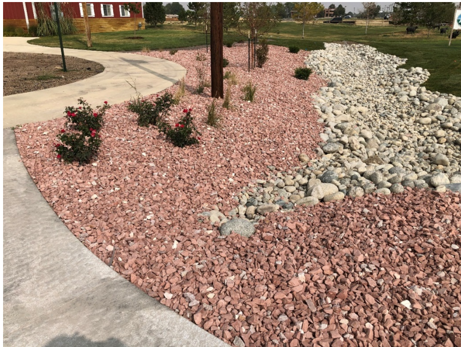
Storm drainage integrated with landscaping, lawn in background. Steve Hebert photo, Town of Bennett Planning Department
