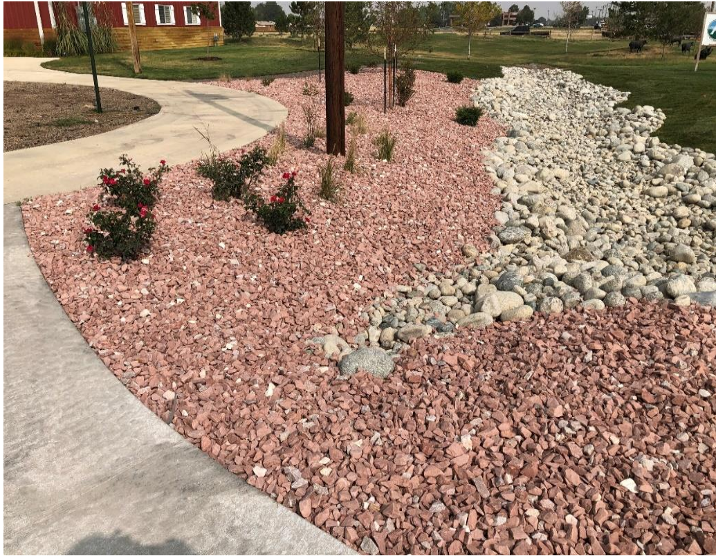
Storm drainage integrated with landscaping, lawn in background. Steve Hebert photo, Town of Bennett Planning Department
