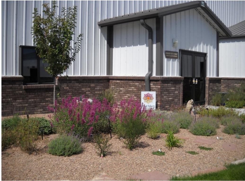
Holyoke Events Center Steve Hebert photo, Town of Bennett Planning Department
