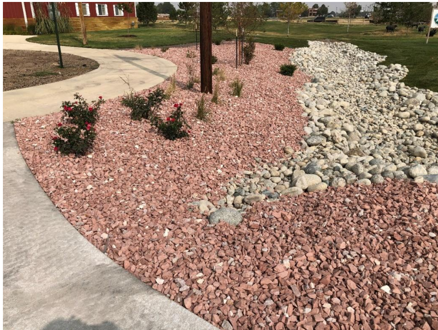
Storm drainage integrated with landscaping, lawn in background. Steve Hebert photo, Town of Bennett Planning Department
