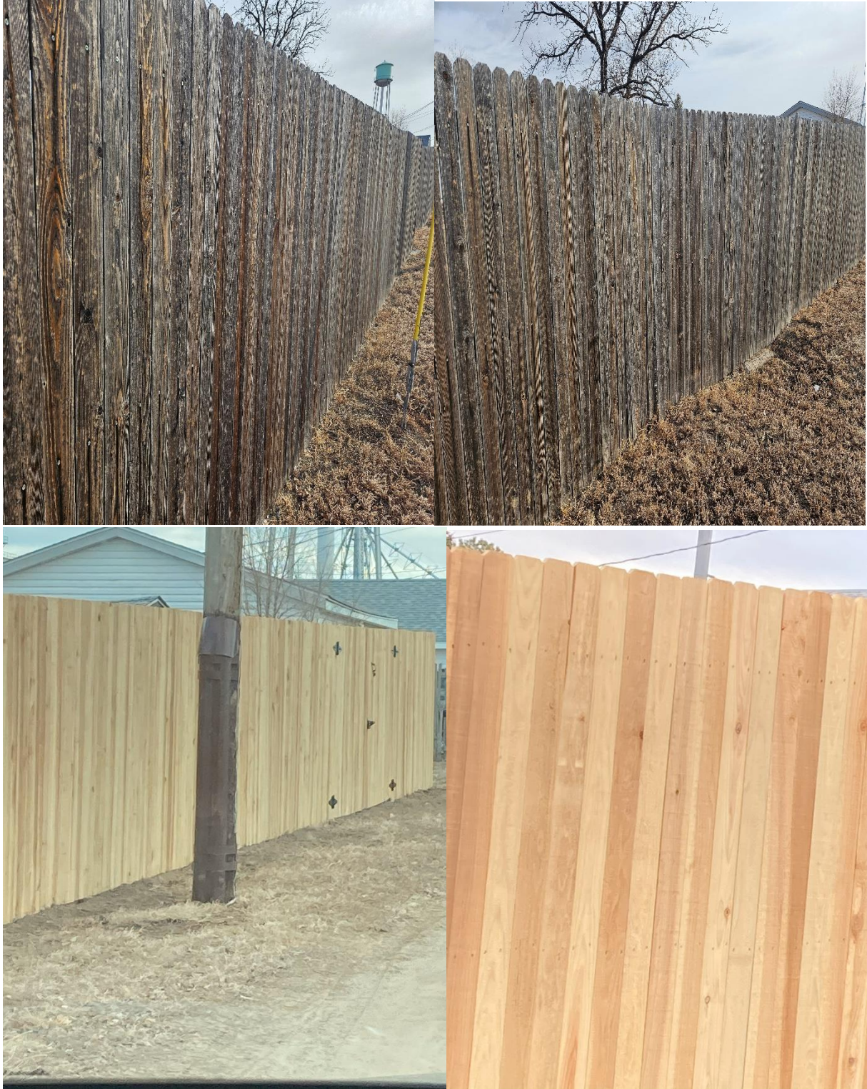
REVIVE Grant New Fencing
