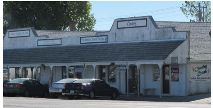
Figure 5.1 Existing Old Town Architecture
